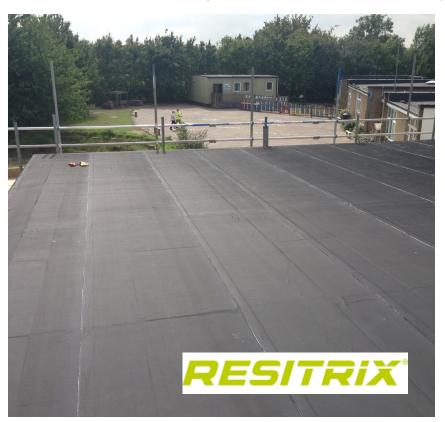
orking with the Main Contractor, B J Davis Ltd of Southend-on-Sea, we completed the overlaying of the new flat roof onto the contractors prepared Plywood roof decking. The ideal product for this type of roof was Resitrix Elastomeric EPDM membrane.
